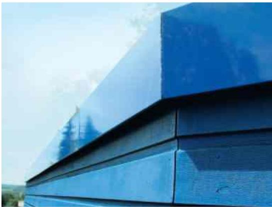
Fig. 1: Facade of a building with polyester powder coating.
