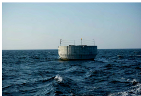
Fig. 8: Offshore anchored concrete foundation
