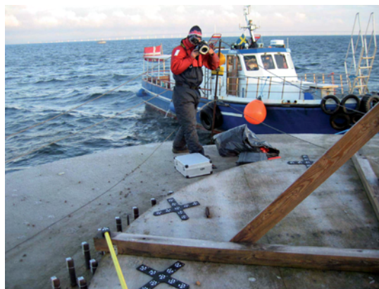
Fig. 10: Measurement and inspection of 120 mounting bolts with the TRITOP CMM system on high seas
