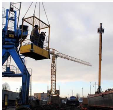
Fig. 6: Mobile measurement of the complete hull with the TRITOP CMM system.
